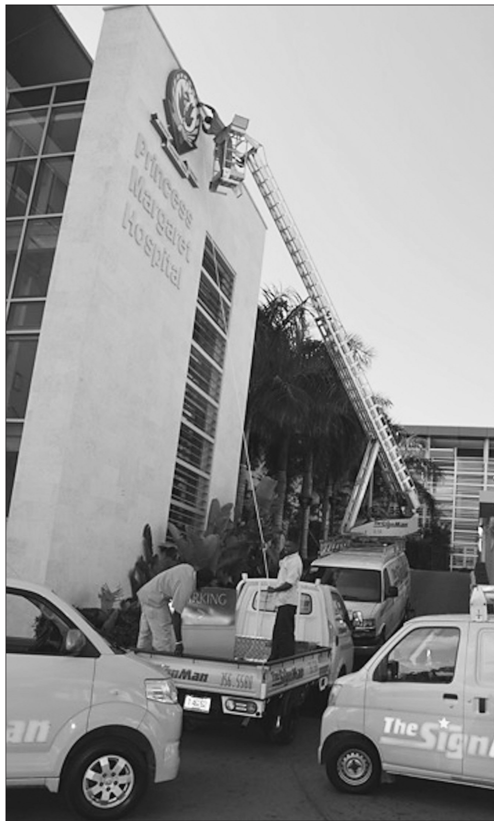
SIGNMAN workers installing new signage at the Princess Margaret Hospital.
